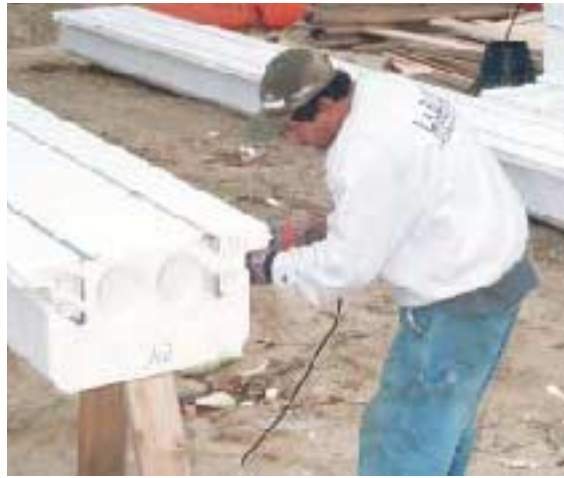
Figure 7. The 24-foot-long panels were shortened to bear only on the inner edge of the foundation forms. A recip saw was used to cut through the integral steel Z-beams. The entire 24x36-foot deck was covered within an hour.
