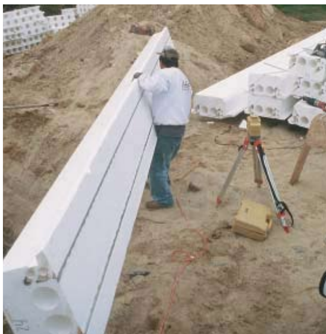
Figure 1. At roughly 2 pounds per linear foot, the interlocking deck panels can be carried and set in place by a single worker with relative ease.
