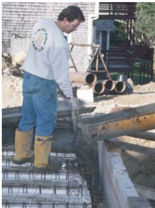
Figure 13. A triangular wood screed strip attached to the wall form guides the thickness and slope of the floor and provides a beveled edge to the finished slab (left). Below are two views of the project after completion.
