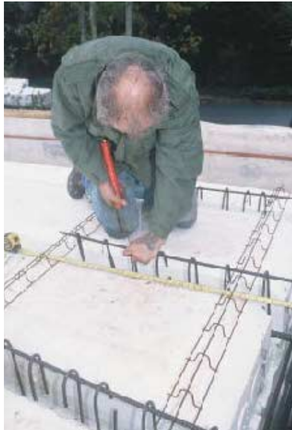
Figure 9. To eliminate a moment connection, steel rebar connecting the floor system to the walls was installed independent of the wall rebar, providing for possible movement in the floor to be released at the top of the wall (left). The right-angle connecting rods were tied to the #8 longitudinal rod with #2 rebar stirrups, placed 5 inches on-center over a 3-foot run (below).
