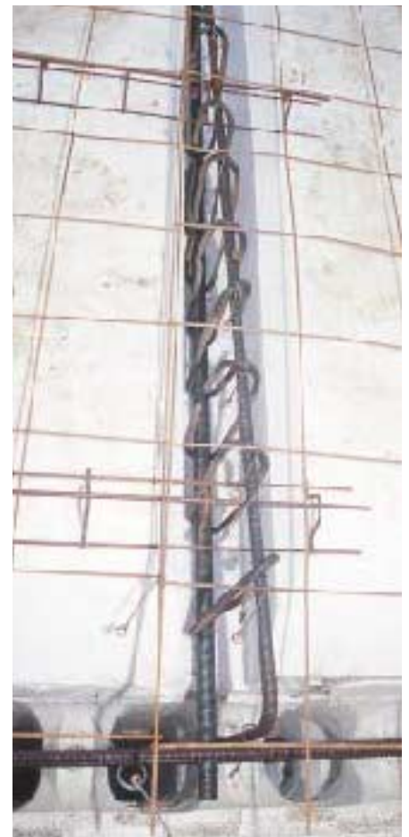
Figure 9. To eliminate a moment connection, steel rebar connecting the floor system to the walls was installed independent of the wall rebar, providing for possible movement in the floor to be released at the top of the wall (left). The right-angle connecting rods were tied to the #8 longitudinal rod with #2 rebar stirrups, placed 5 inches on-center over a 3-foot run (below).
