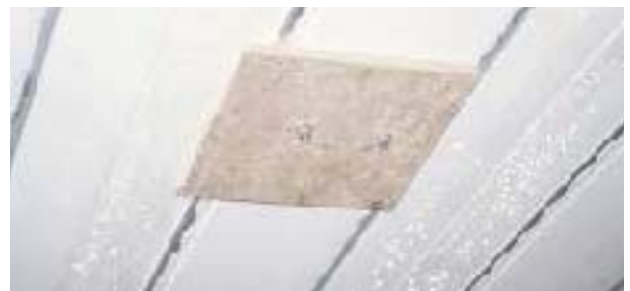
Figure 11. To provide for a chain fall or hoist, the author installed a pair of foundation anchor bolts through one of the floor forms. The bolts are set in a cavity scooped out of the deck form and tied to rebar extending back to two adjacent joists. The bolts will be used to attach a rugged bracket to the ceiling below.
