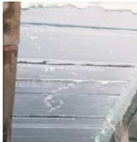
Figure 12. The pressure generated by vibrating and compacting the concrete began to force pieces of retrofitted foam blocking out of place, despite the use of foam adhesive. Backing off on the vibration averted a blowout.
