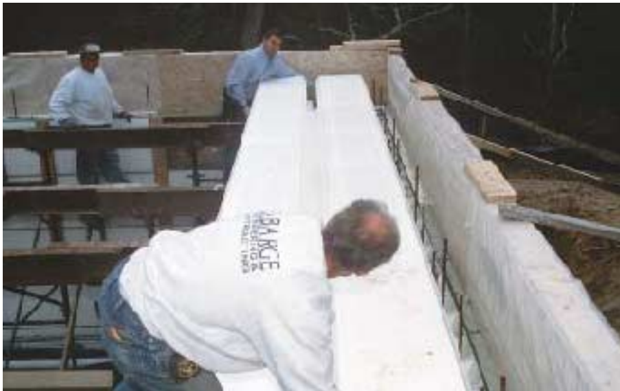
Figure 7. The 24-foot-long panels were shortened to bear only on the inner edge of the foundation forms. A recip saw was used to cut through the integral steel Z-beams. The entire 24x36-foot deck was covered within an hour.
