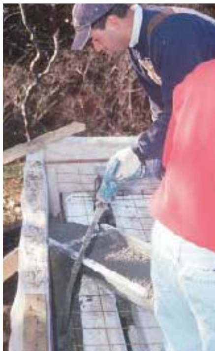
Figure 12. The pressure generated by vibrating and compacting the concrete began to force pieces of retrofitted foam blocking out of place, despite the use of foam adhesive. Backing off on the vibration averted a blowout.
