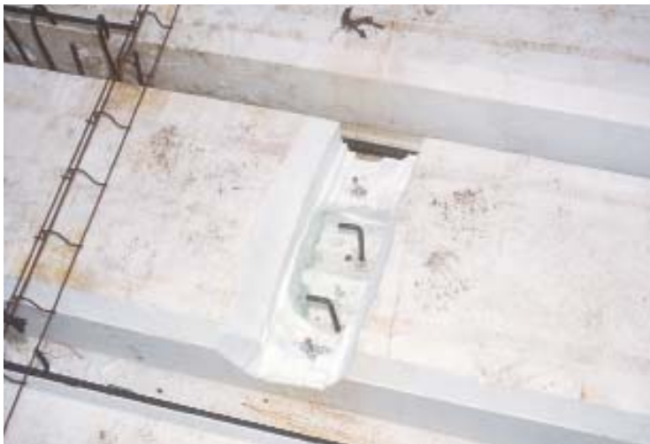
Figure 11. To provide for a chain fall or hoist, the author installed a pair of foundation anchor bolts through one of the floor forms. The bolts are set in a cavity scooped out of the deck form and tied to rebar extending back to two adjacent joists. The bolts will be used to attach a rugged bracket to the ceiling below.
